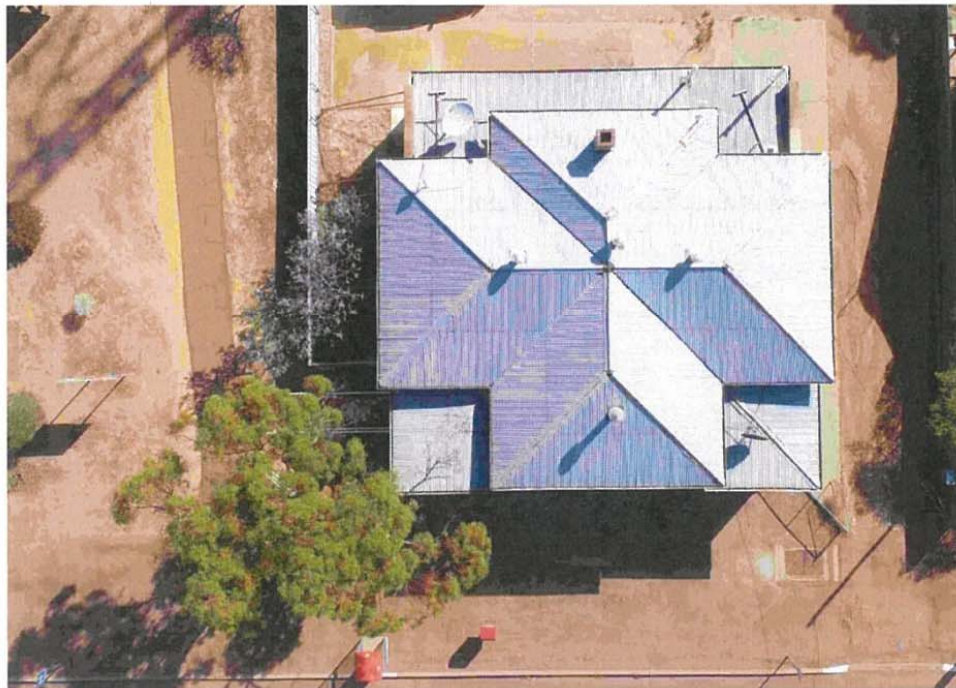
Figure 2: Aerial image of Nungarin post office.
