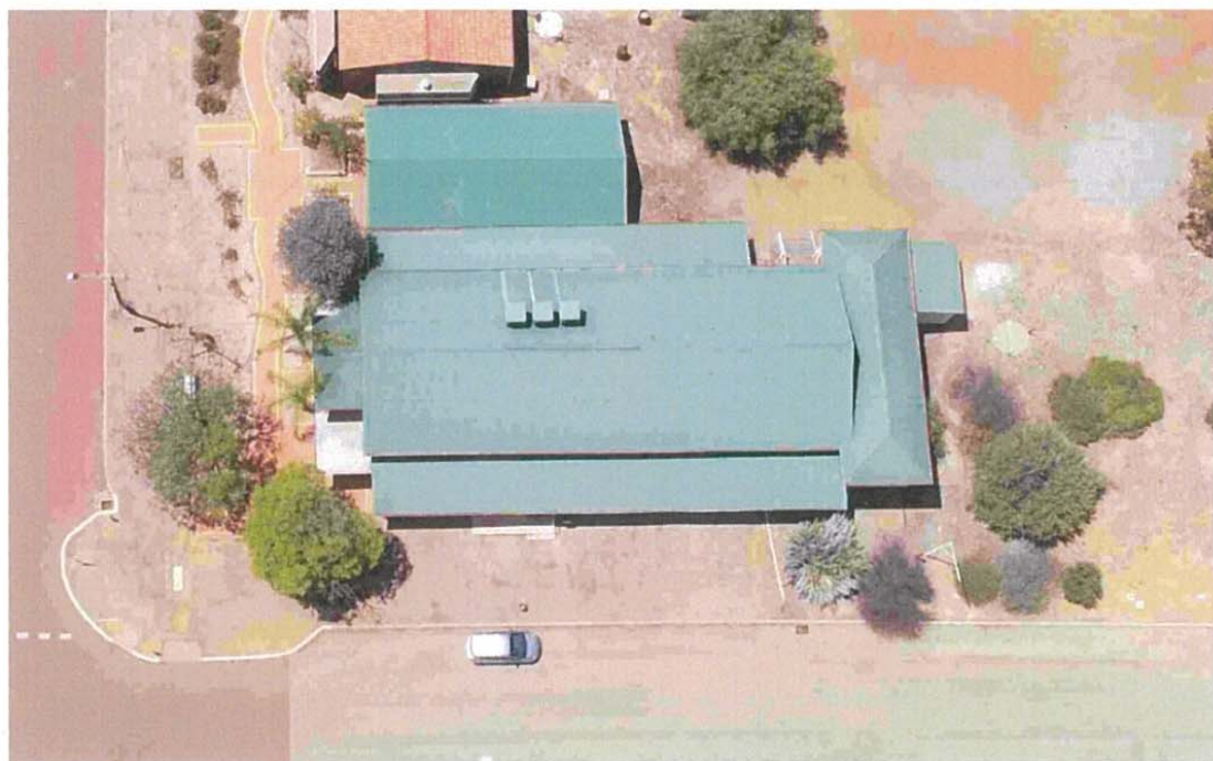
Figure 2: Aerial image of Nungarin Hall.
